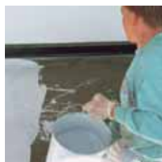
StoPur EB 200 felhordása
